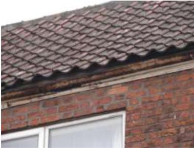
Swifts may nest behind the aperture in the cornice above the right hand window in the photo above. A simple solution is preserve the nest space to cut an aperture in the replacement cornice, (as shown on the right) or to offset the new cornice with battens so the Swifts can enter underneath it.
