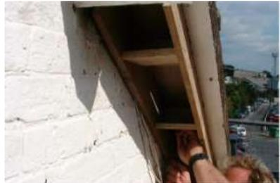
A Schwegler "Swift Brick" inserted into previously open eaves to provide a replacement Swift nesting place. The roof of this NHS hospital had to be sealed to meet hygiene requirements, but the Swifts' nests were saved.
