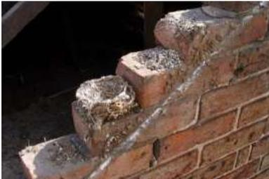
The gable brick ends shown exposed on the left have been fitted with bargeboards containing staircase type nest boxes. These will be faced with a plank with entrance holes cut for the Swifts to access the new nest places inside.
