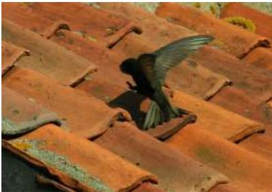
A Swift entering a roof via a displaced pantile. The nest is on the roofing felt below, held in place by the battens. This sort of nest place can be protected by wedging up the replacement tiles wherever the nest entrances are. The access gap needed by the Swifts is just 30mm.
