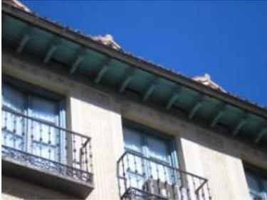
Swifts nest under the tiles on the brick ends of this roof. Repairs would evict them, but leaving the bricks as they are and fitting deeper tiles, offset to maintain the Swifts' access from below, will provide weather proofing and still let the Swifts nest.
