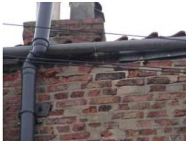
Swifts can often be found nesting in gaps in brickwork behind pipes, flashings and gutters. Great care is needed when replacing these items not to destroy access. The simplest solution is to keep the holes open, place flashing and pipe brackets so as not to obstruct access.
